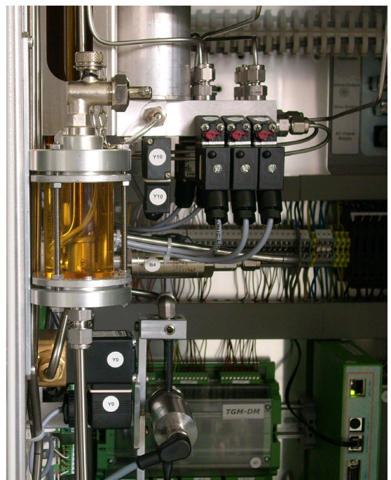
Fig.1 Gas collector for Buchholz gases in TGM
