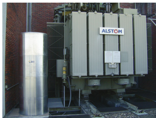
Fig. 2 G3B installation on an industrial transformer
